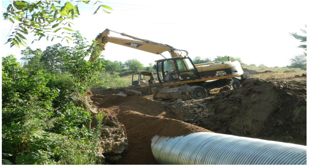
Bill Wiederholt in the excavator, installing a new culvert.
